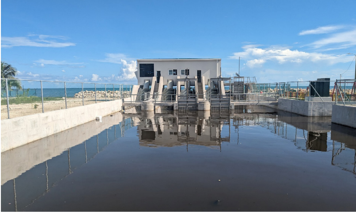
Belize City pumping station. Credit: Natalie Fiertz, October 2023.
