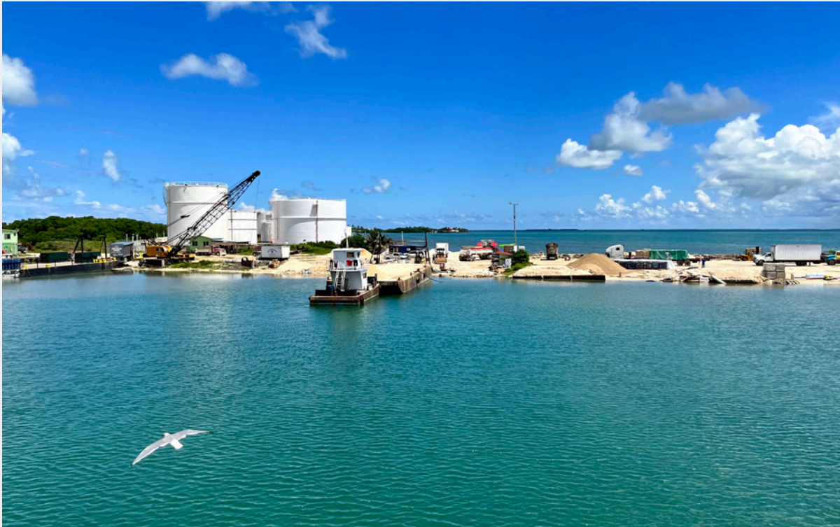
Repairs to the Belize City port. Credit: Carolyn Gruber, October 2023.
