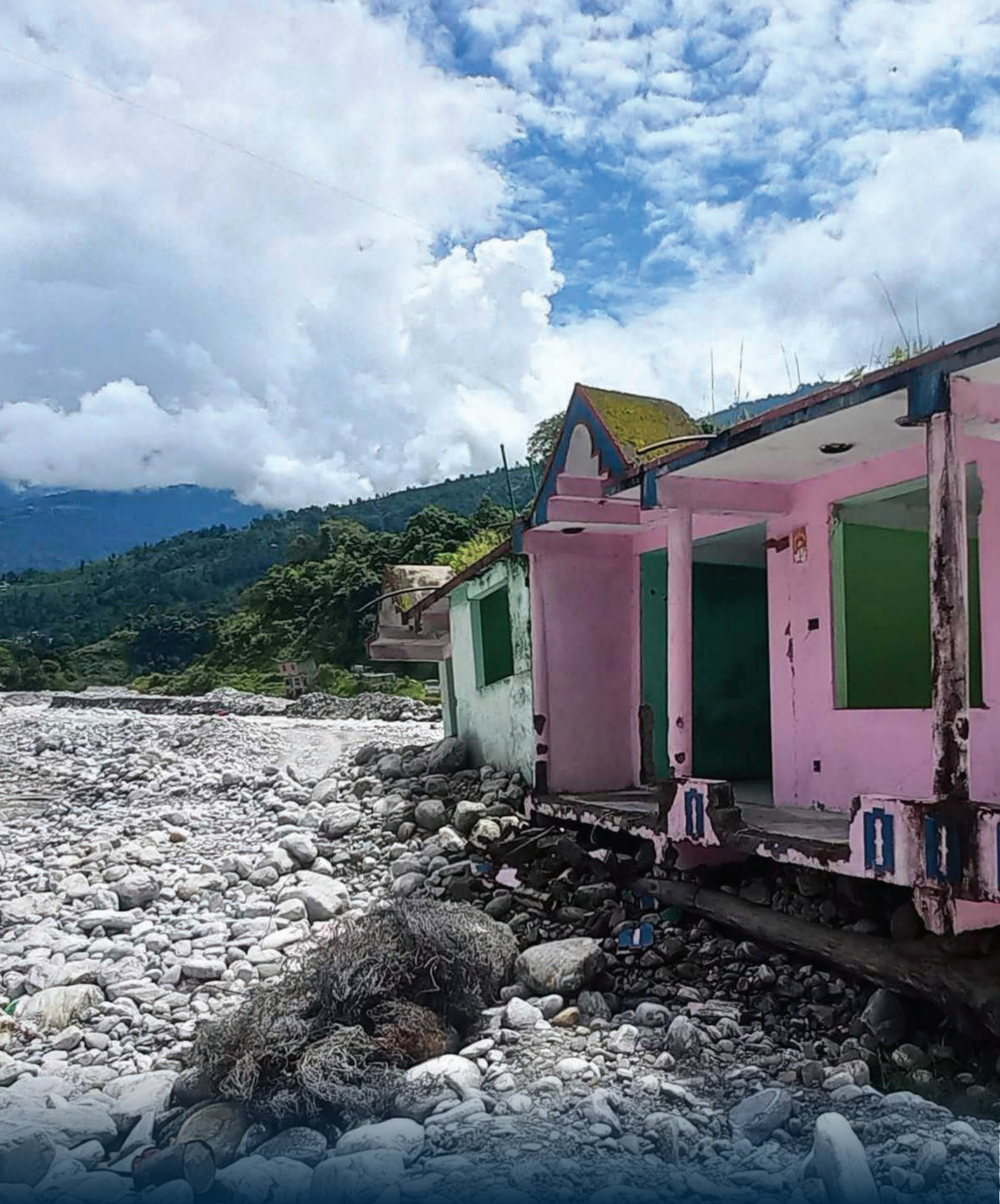
Aftermath of the Melamchi incident. Photo courtesy of Jakob Steiner.
