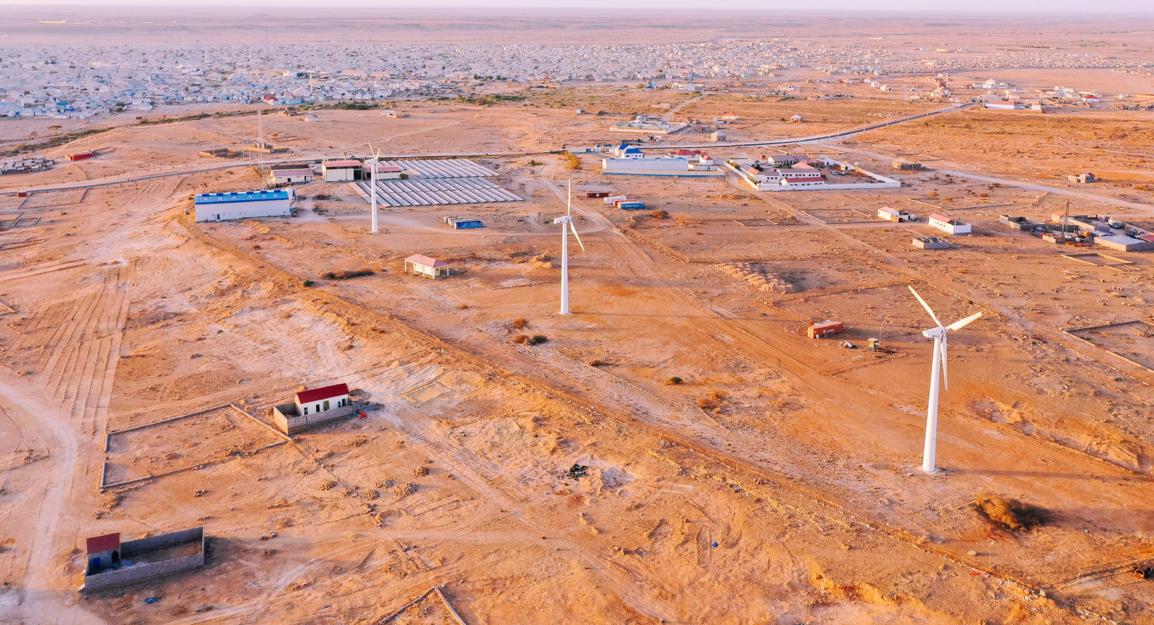
NECSOM Power Plant, Garowe, Puntland State of Somalia Photo: Faaris Adam
