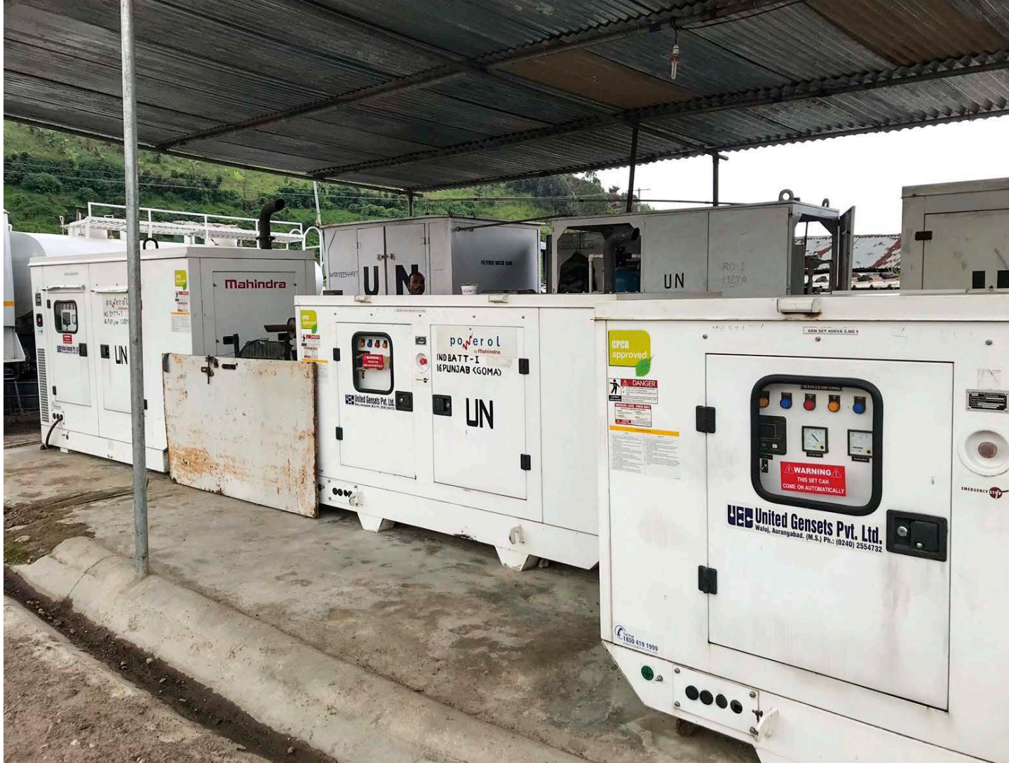
Old generators at the TCC base at Munigi, out of service since the site was connected to hydropower.
